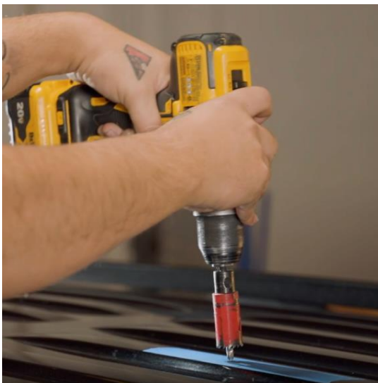
Figure 6 –Drilling the hole.
